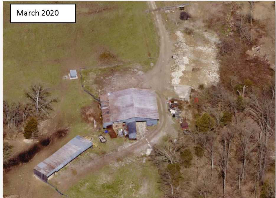
Aerial showing fill being placed on the site which later became the equipment parking and staging area.
